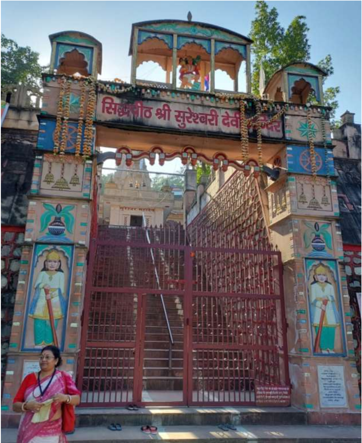
MAIN GATE OF SHRI SURESHWARI DEVI TEMPLE, RAJA JI NATIONAL PARK, HARIDWAR
